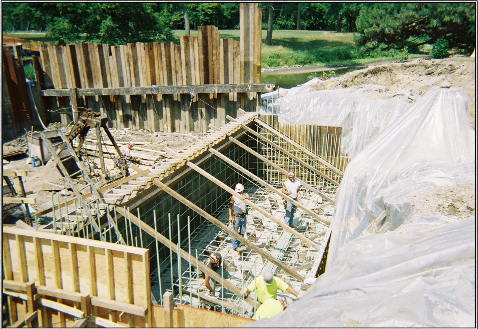
Placement of Bar Steel Reinforcement for the east abutment. Please also note the dry condition of the cofferdam. The cofferdam was required, per the WDNR, so a concrete sill, present beneath the original structure, could be removed under dead water conditions.
