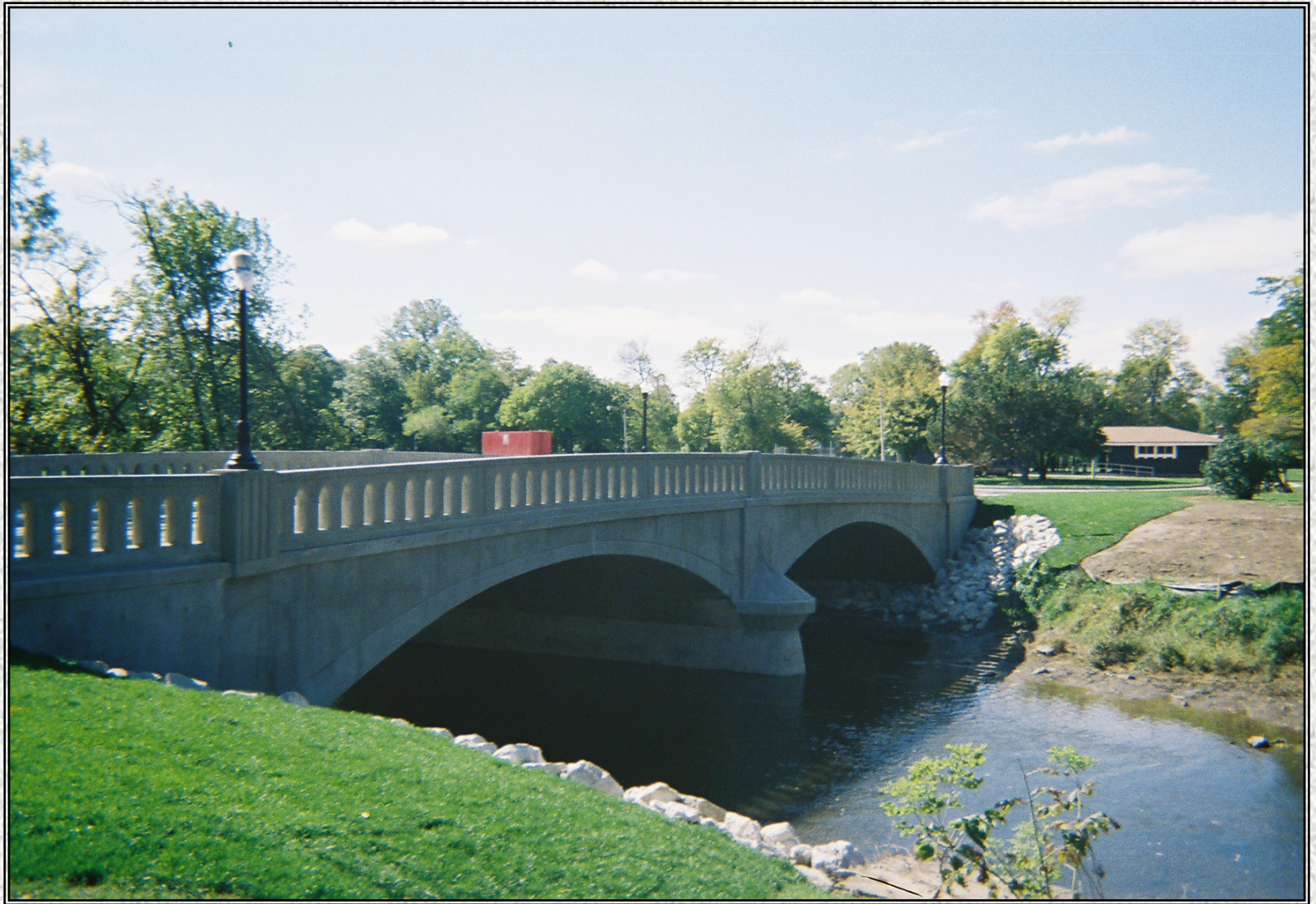
View of the completed structure (B-51-108) from the Northeast.
