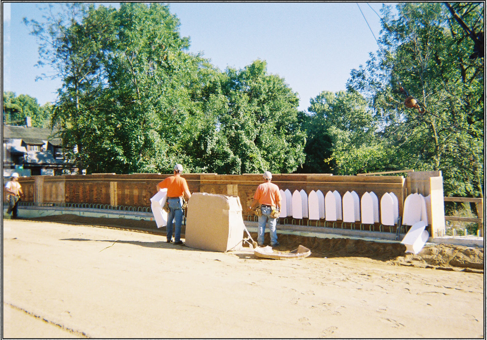
Layout and forming of the South parapet wall on Bridge B-51-108.
