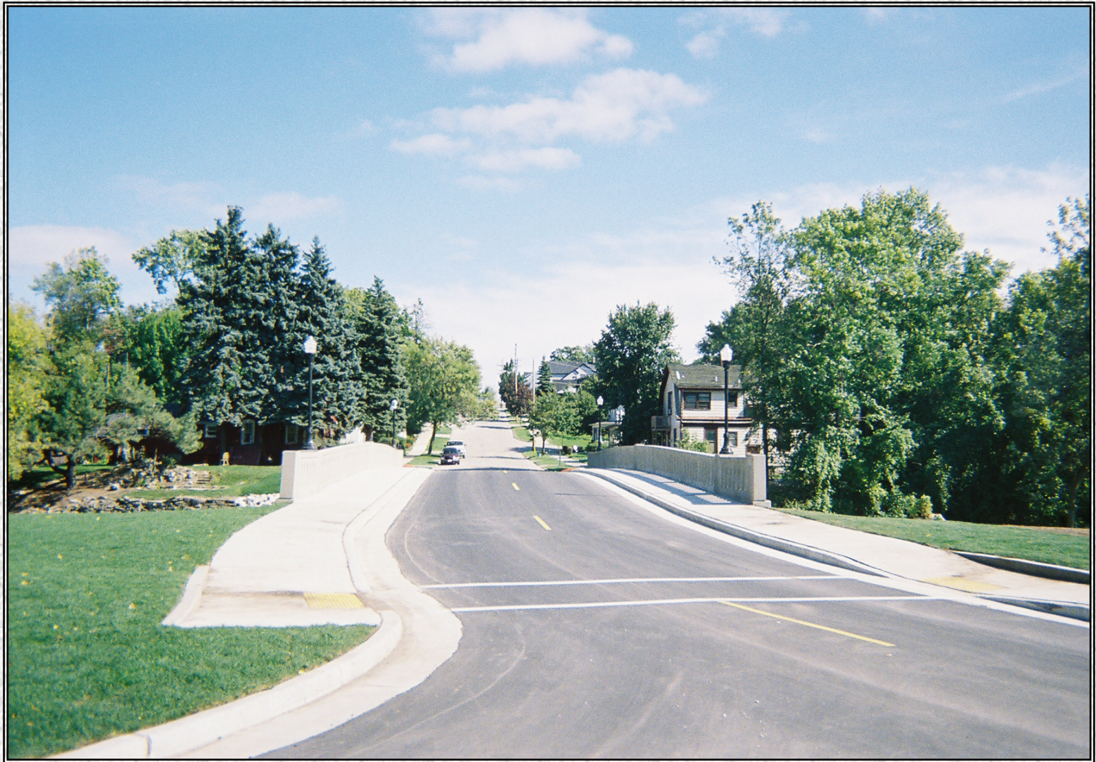
View of the newly completed roadway and bridge (B-51-108) from Island Park, Racine, Wisconsin
