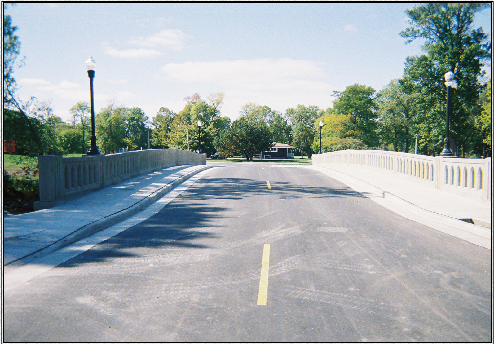
Looking West into Island Park over the newly completed bridge (B-51-108) and roadway.
