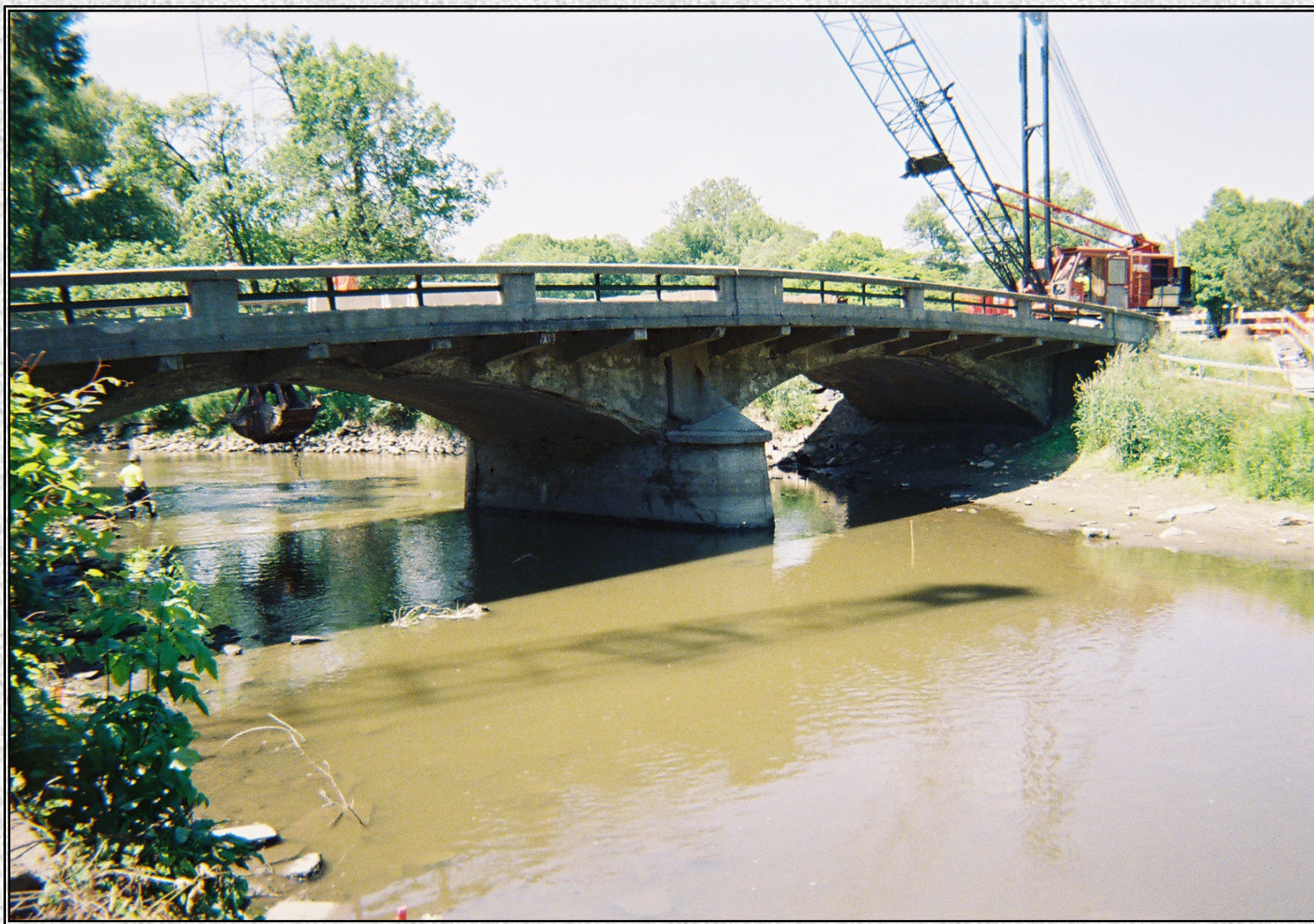
Looking South toward the original structure prior to bridge replacement.
