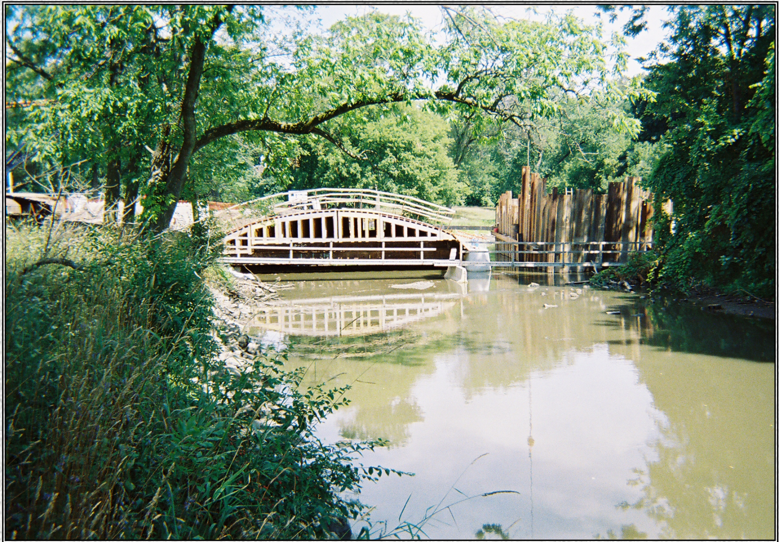
Looking upstream at the falsework for the western spandrel arch and the WDNR mandated cofferdam for east abutment construction.
