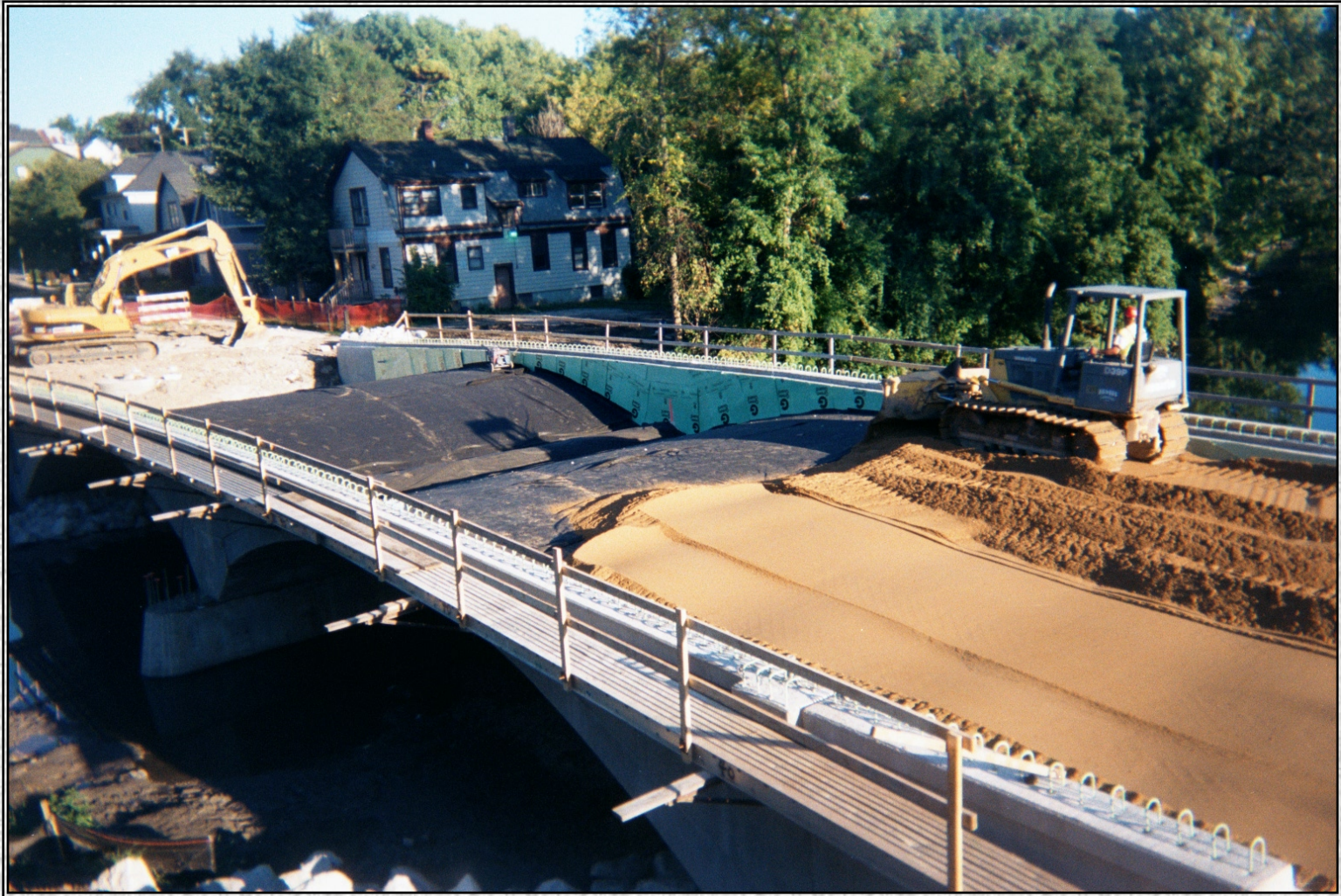
Placement of structure backfill over the superstructure following installation of the waterproof membrane. Liberty Street Bridge B-51-108
