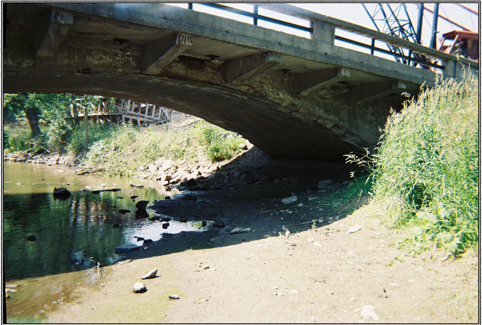
Underside view of the original structure prior to bridge replacement.
