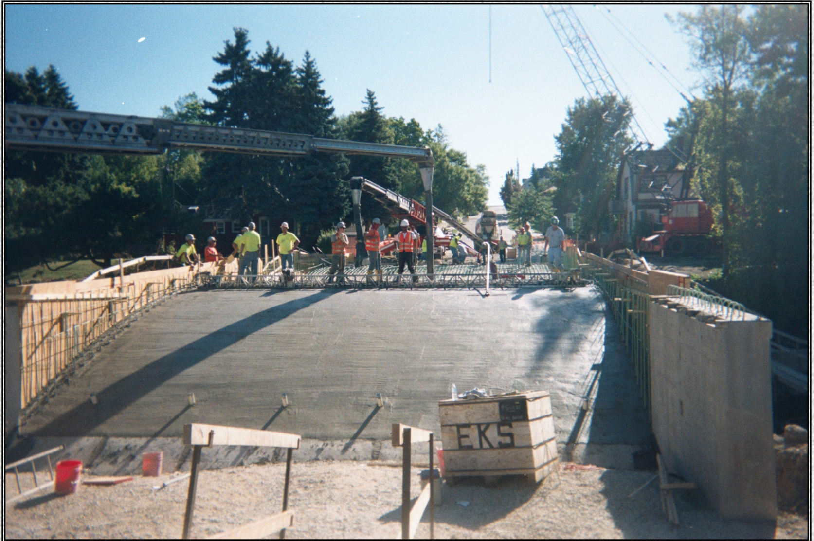
Completion of the deck pour on Structure B-51-108. Please note that the quality of the finished surface allows for better adherence of the waterproofing membrane.
