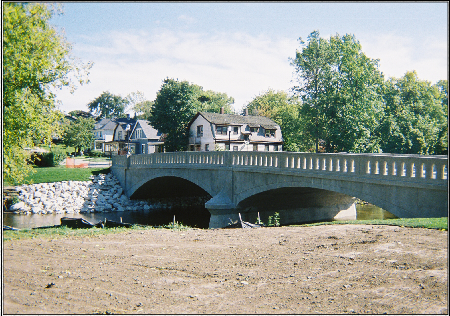
View of the completed structure (B-51-108) from the Northwest.
