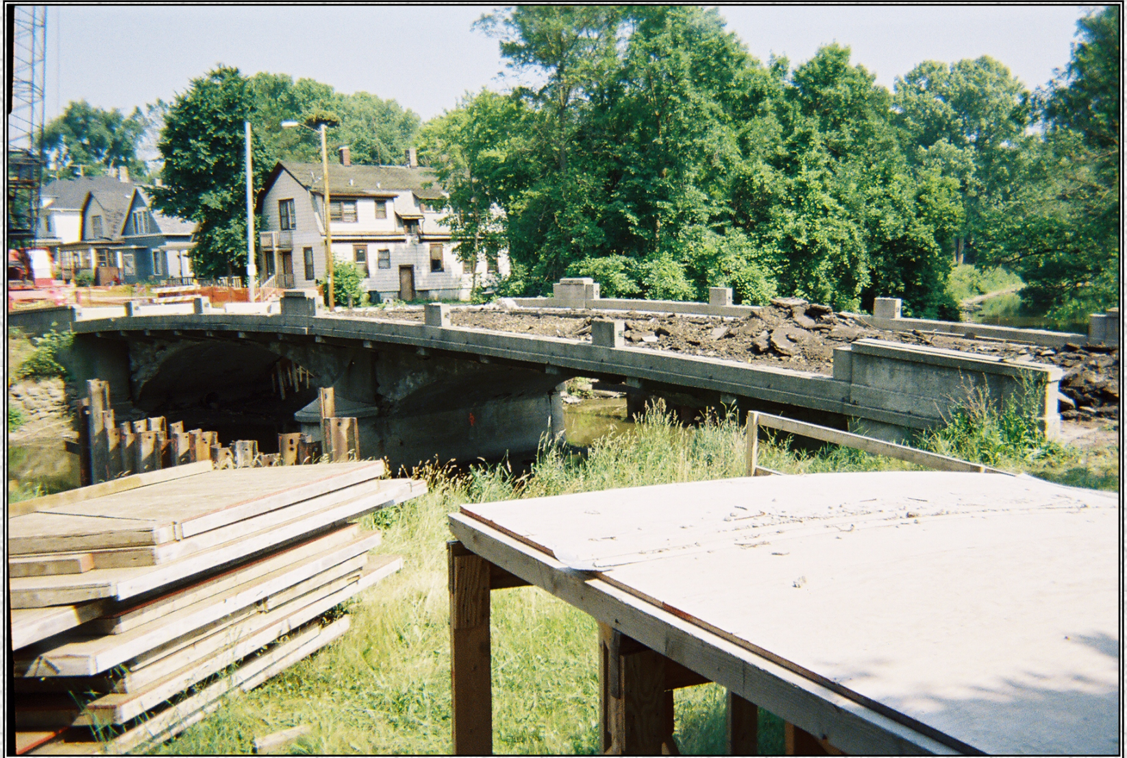
Removal of earthen fill from the original bridge was performed within the footprint of the original structure and performed in a manner to prevent sediment discharge into the underlying Root River.
