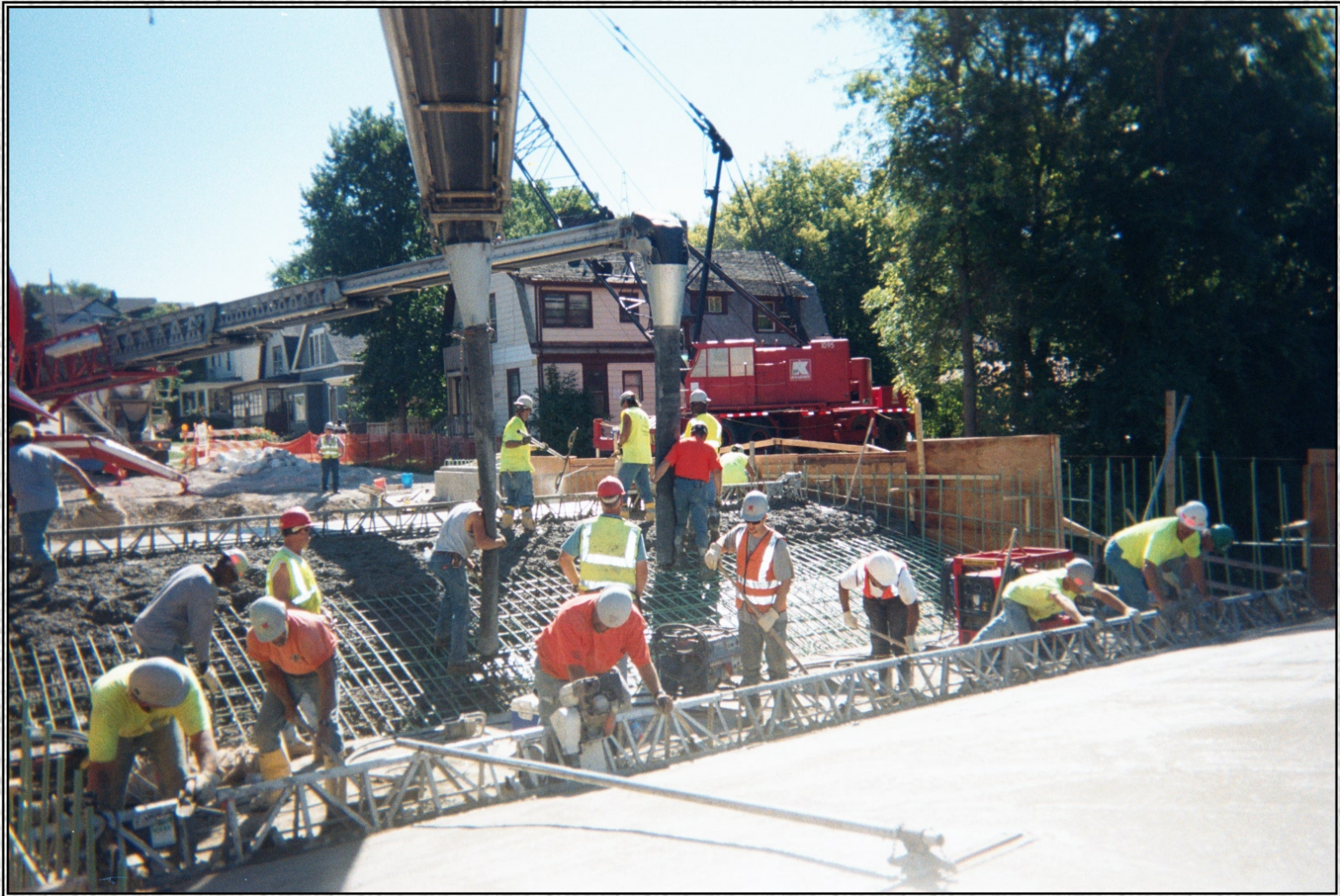
Pouring the superstructure on Bridge B-51-108. Edward Kraemer & Sons used 20 individuals to pour the twin spans. Conveyor trucks on each side of the bridge delivered concrete to the deck.
