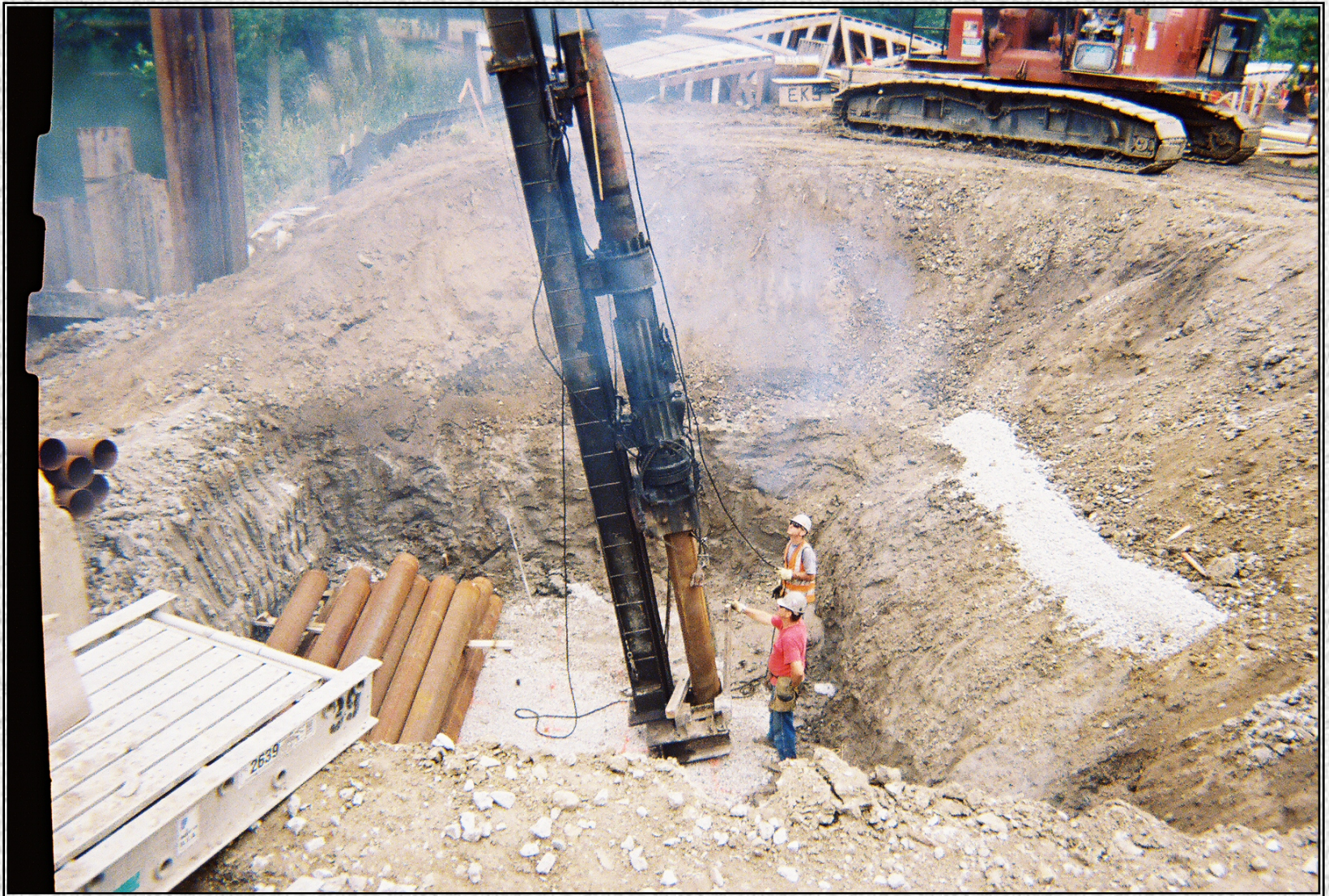
Driving Cast in Place Concrete Piling on the West Abutment of Structure B-51-108. Please note the 1' in 4' batter on the piling.
