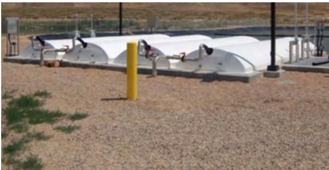
Figure 11-15. Example Half-Barrel Cover Installation
