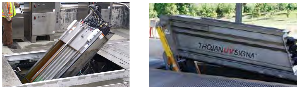
Figure 11-14. Signa UV Lifting Systems (2R left; 4R right)
