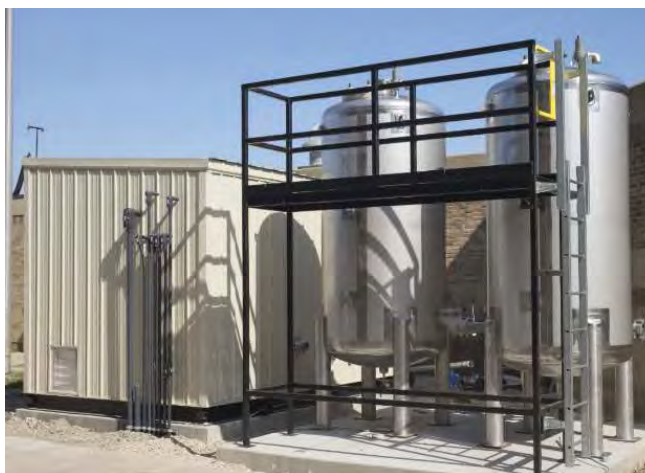
Figure 11-27. Hydrogen Sulfide Treatment Vessels
