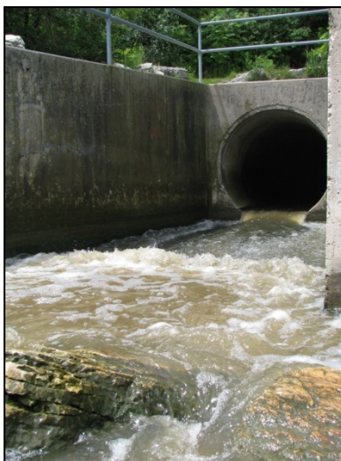
Figure 1: Wolff Street Outfall at south end of Michigan Boulevard Beach
