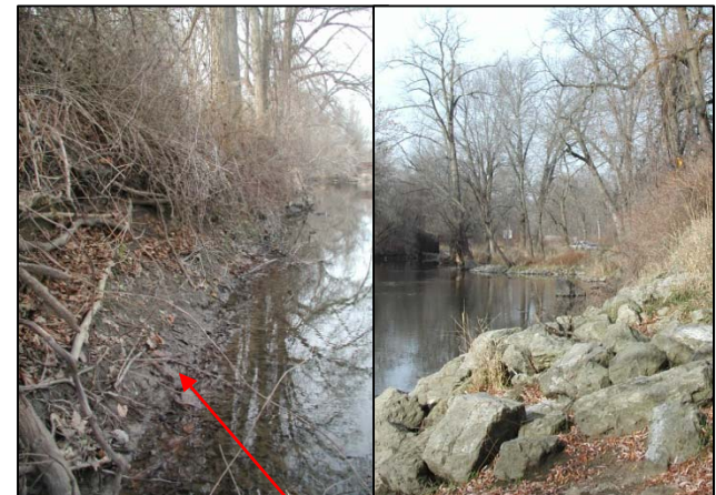
Steep eroded banks (left) at the foot of a bluff with residences on west bank and free-standing rock pilings on east bank next to park (right).
