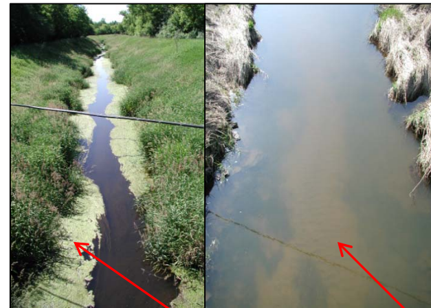
Accumulation of high algal growth (left) and fine sediment in canal bed (right).
