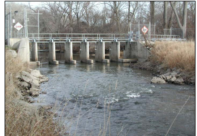
Looking downstream from sampling location in winter. Fish weir runs across stream width and free-standing rocks stabilize nearby banks.
